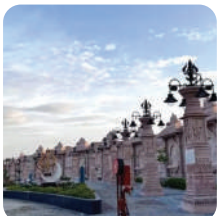
MAHAKAL LOK CORRIDOR
